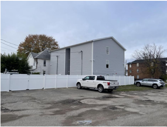
View of the rear of the building from the east side of 15 th street. Automobiles in this picture are parked in the right-of-way.
