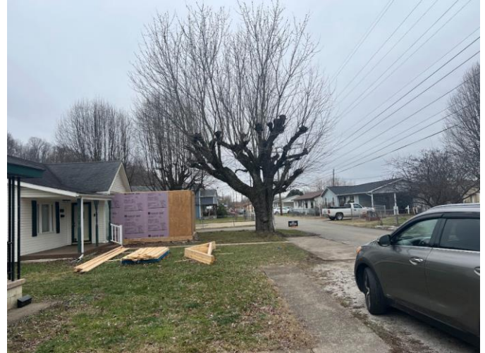
View of petitioned property looking west on Bradley Road.
