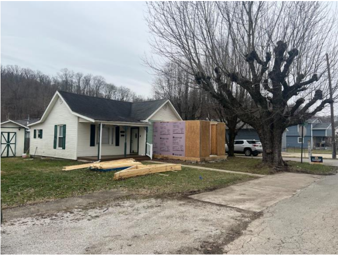
View of petitioned property looking southwest from Bradley Road.
